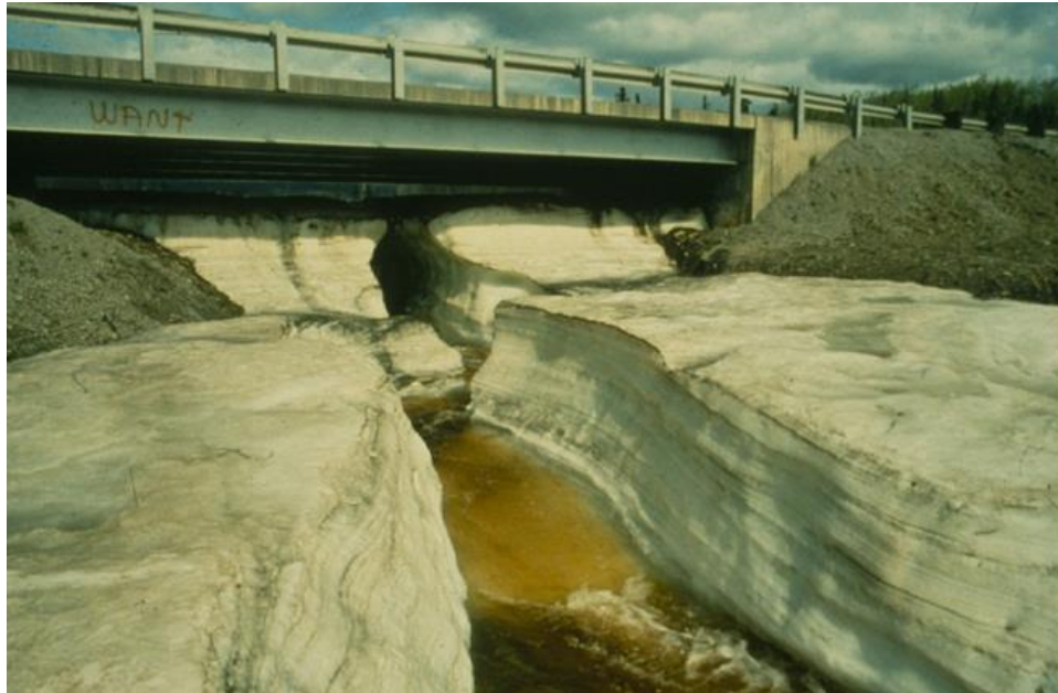
Figure 4.1.1-7: Aufeis at a Bridge Near Fairbanks, Alaska
