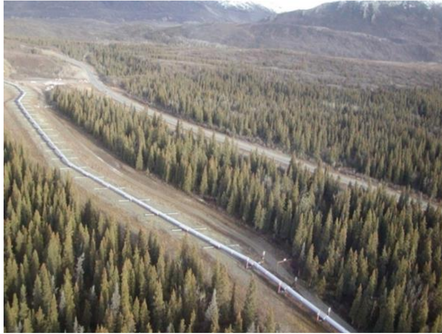
Location where Trans-Alaska Pipeline System crosses the Denali fault (2012). Note how pipeline shifted to left of center on the Teflon-coated beams. Source: USGS 2012.
