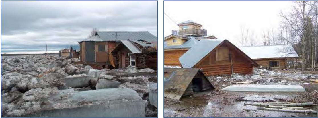
Flooding due to the 2009 spring ice jam floods on the Yukon River. Source: DHS&EM 2009.
