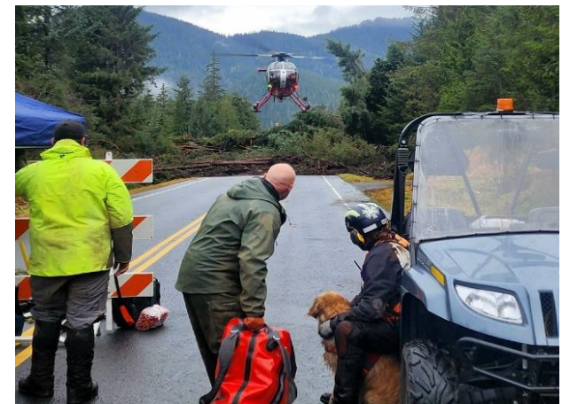
Wrangell, Zimovia Hwy., Landslide 2023
